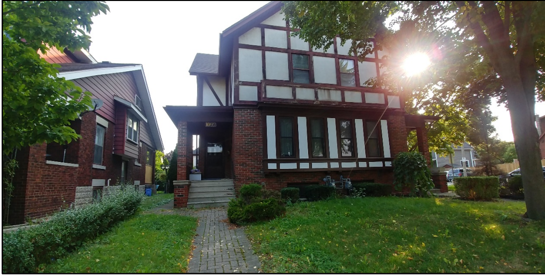
Figure 1b – Street View – Dougall Ave (Source: Pillon Abbs Inc)
